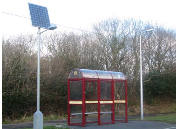
Examples of Photovoltaic Installations in the Carmarthenshire Street Scene
